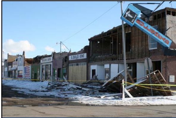
Wells old town after the earthquake
